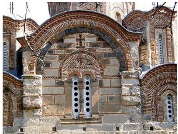
4a. St. George, western facade bifora
